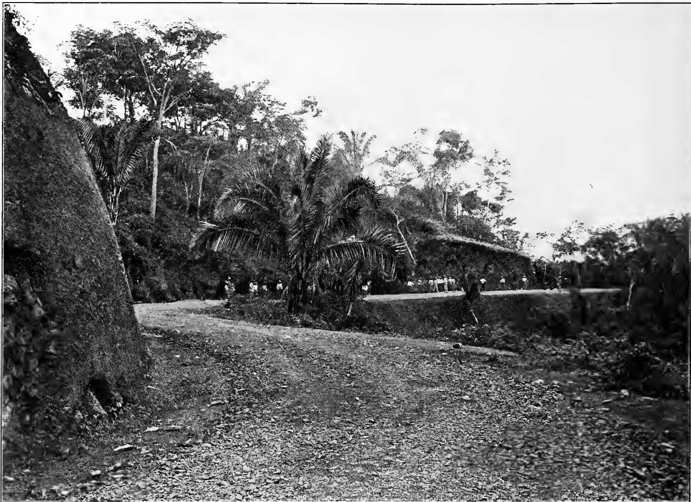
CONVICTS BUILDING A COMMISSION ROAD
